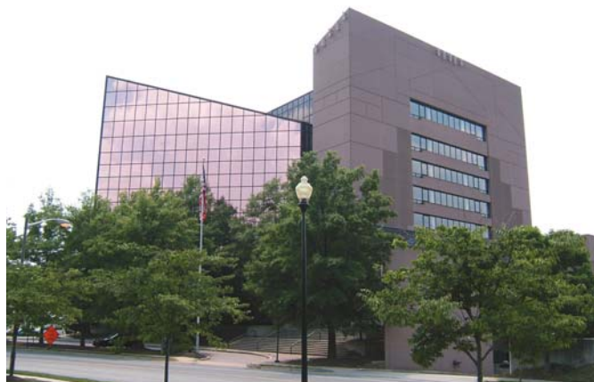
ATA's building on 2200 Mill Road.
