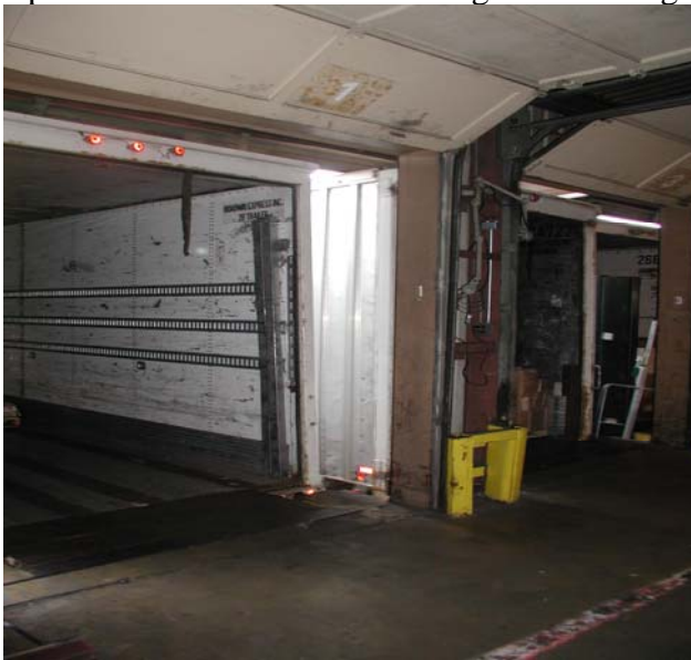
(Interior of trailer at dock - note the minimal gap between the side of the trailer and the dock bay opening)
